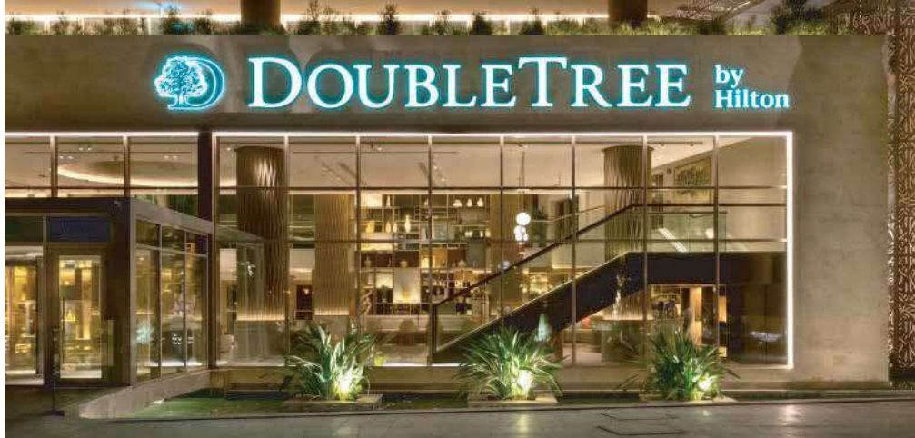
DOUBLETREE BY HILTON EI GOUNA Lighting
