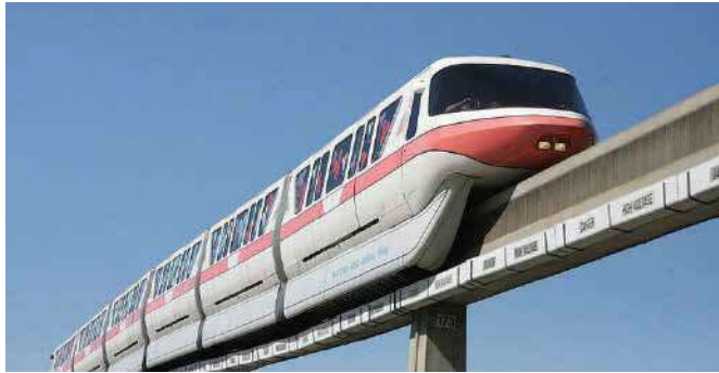
MONORAIL- OCTOBER Cable Trays
