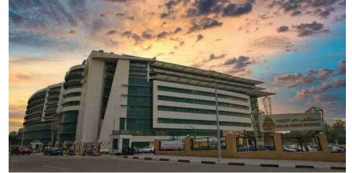
DAR EL FOUAD HOSPITAL Bus Trunking System
