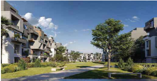
SODIC-EAST-NEW-CAIRO-COMPOUND Lighting Poles
