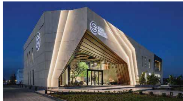
SAUDI EGYPTIAN DEVELOPERS Indoor + Outdoor Lighting Design
