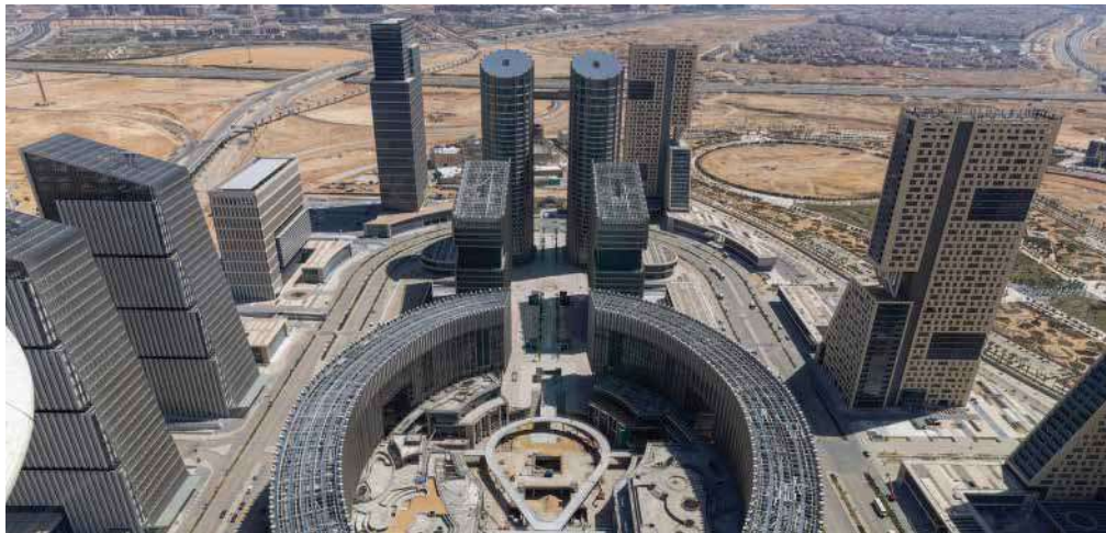
CBD CENTRAL BUSINESS DISTRICT - NEW CAPITAL Cable Trays
