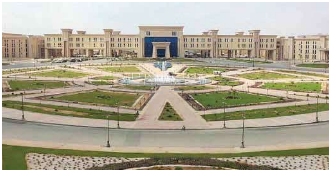
THE OCTAGON BUILDING Cable Trays
