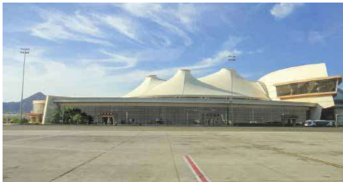
SHARM ELSHEIKH AIRPORT Power
