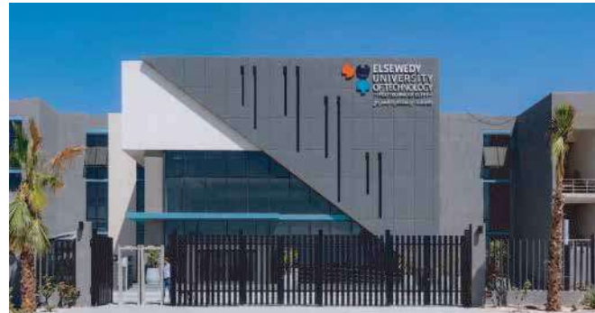
ELSEWEDY UNIVERSITY OF TECHNOLOGY Indoor Lighting
