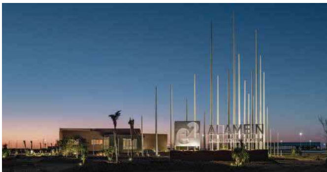
ALAMEIN INDUSTRIAL PARK Outdoor Lighting
