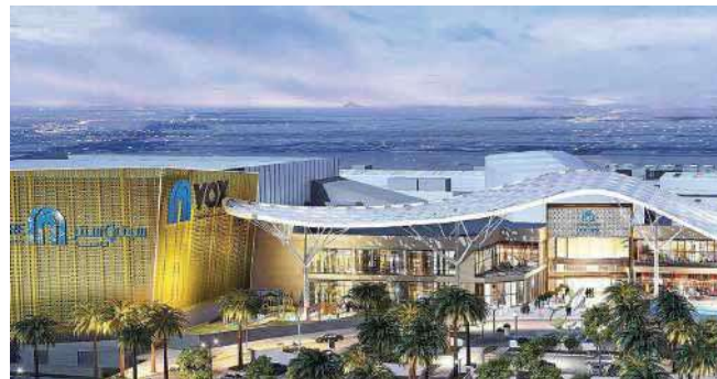
THE ALMAZA MALL ALFUTTAIM GROUP Cable Trays
